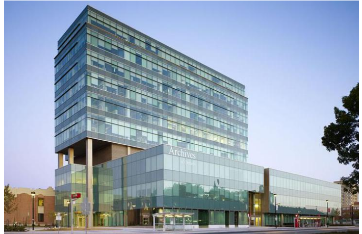
Setbacks from base buildings reduce the visual and physical impact of taller elements including wind and shadowing conditions (Research Tower, York University).
