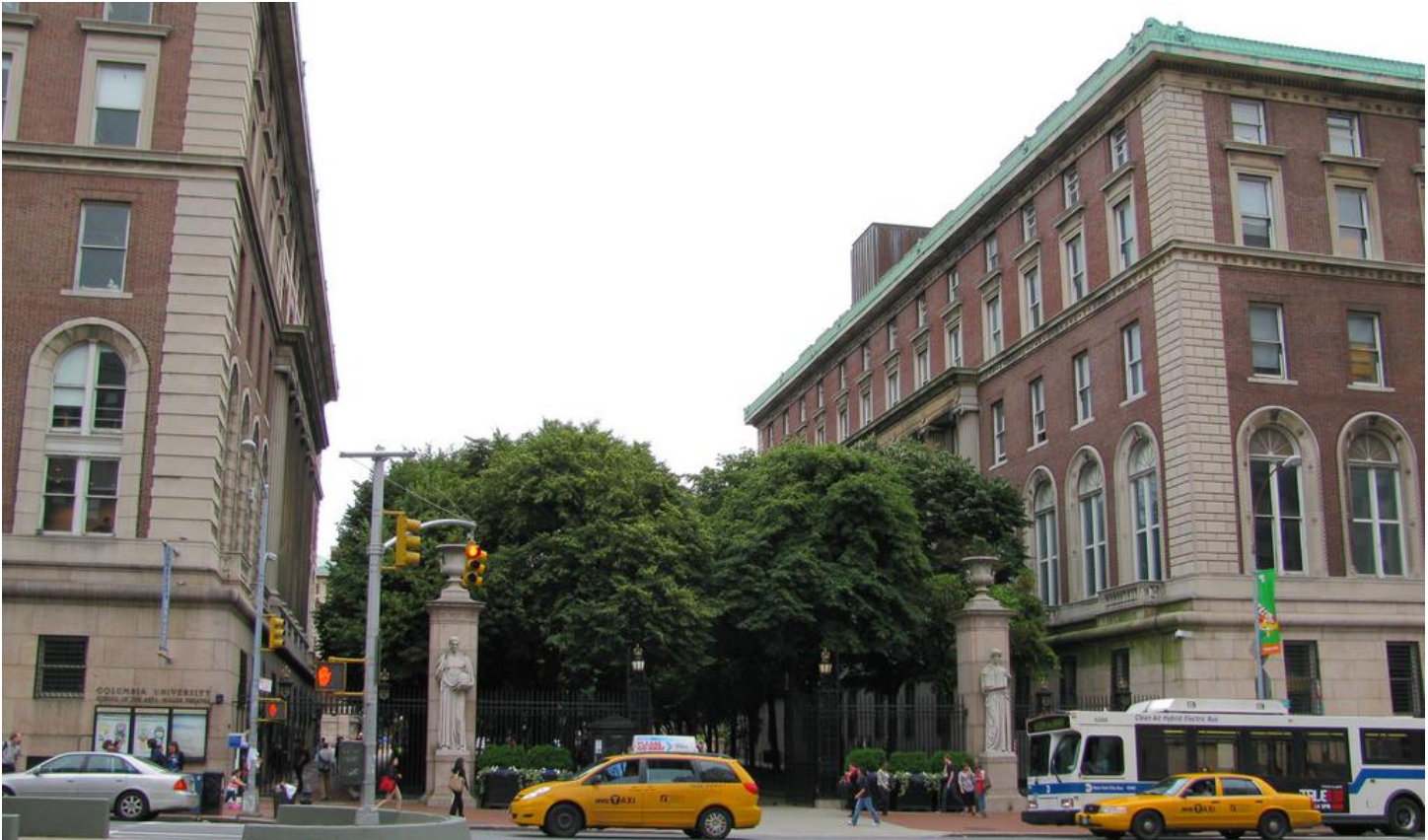
Traditional gateways often incorporate symmetrical built form and landscaping features.(Columbia University, NY).
