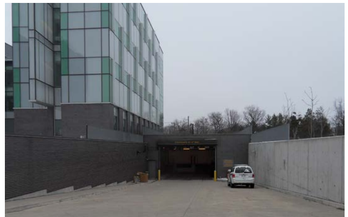
Combined service and loading areas reduce overall building footprints and minimize visual impact on the public realm (combined Instructional Centre and ESCB Loading Area, UTSC).
