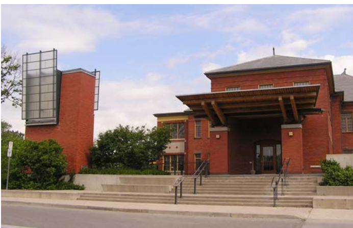
Recessed and covered entrances support more comfortable wind conditions at-grade (Humber River College, Toronto, ON).
