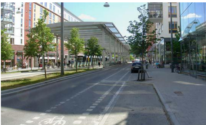
Landscaping and lay-by parking create clear demarcations between multi-modal travel lanes (Hammarby Sjöstad, Sweden).
