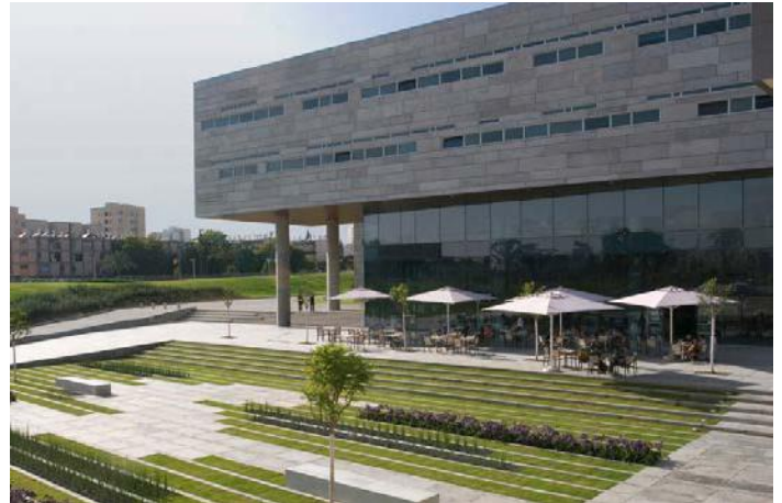
Cantilevers and transparent glazing support a more permeable interface between buildings and adjacent open spaces (Ben-Gurion University, Israel).
