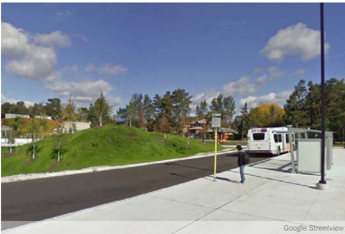
Low-impact stormwater management features can be integrated into transit waiting areas to support a more attractive and sustainable campus. (Highland Hall Bus Loop, UTSC).
