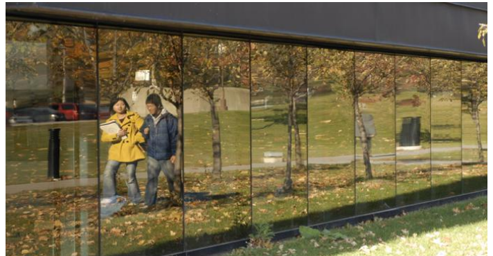
Where non-active uses are contemplated, reflective glazing at grade encourages a sense of permeability and interaction between indoor and outdoor spaces. (Academic Resource Centre, UTSC).
