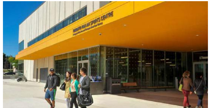
Covered entrances shelter pedestrians from weather conditions and help to indicate primary building access points. (TPASC, UTSC).
