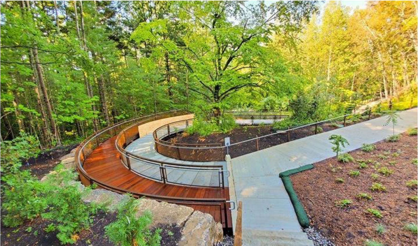
Improvements to Ravine infrastructure provide benefits for all-season use and general accessibility (UTSC).
