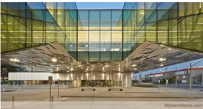
Reflective materials can be used to brighten environments that may have limited access to sunlight (Centennial College, Toronto, ON).
