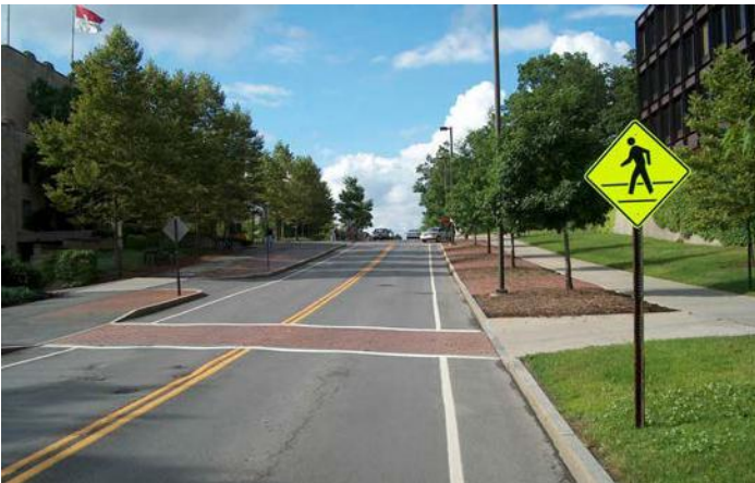
Marked crossings featuring signage and distinct paving support greater pedestrian safety (Cambridge, MA).
