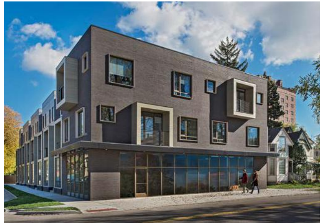
Low-rise, apartment buildings can also provide opportunities for mixed-uses at grade. West Village - Detroit, Michigan
