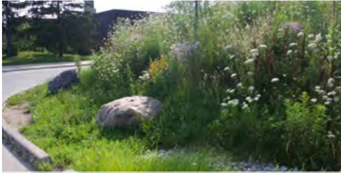
Integrated curb cuts direct runoff from street into adjacent planting
