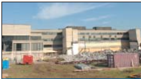
Construction begins on the ARC, scheduled opening Summer 2003.
