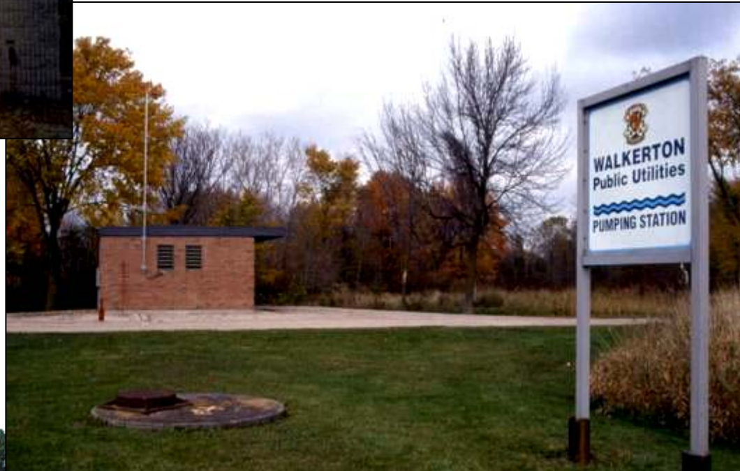
← Well #7, 1986 the deepest (76.2m ) and “main well” producing 3400 litres per minute of normally good quality water.
